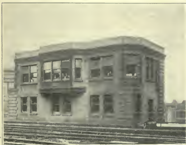
FIG. 290. INTERLOCKING PLANTS. Lake Street interlocking tower of the Chicago & North Western Railway. This is the largest plant of its kind in Chicago.
